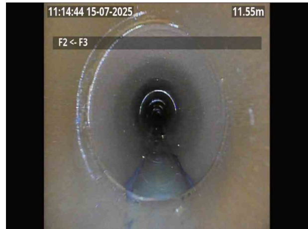
F2X_24fa8d23-09b1-47c7-b50d-393e81cf9de0_20250715_162613_033.jpg, 00:00:59, 11.55 m Fracture, circumferential at joint from 7 o'clock to 12 o'clock
