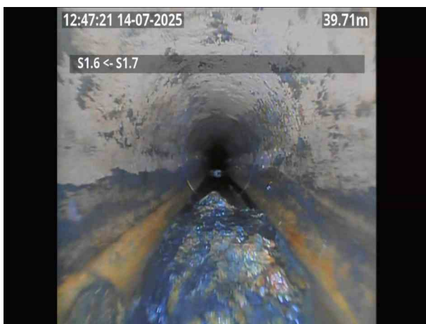
S1.6X_73176655-aae3-438f-b26c-d793b7841327_20250715_134357_875.jpg, 00:03:03, 39.74 m Settled deposits, hard or compacted, 20% cross-sectional area loss
