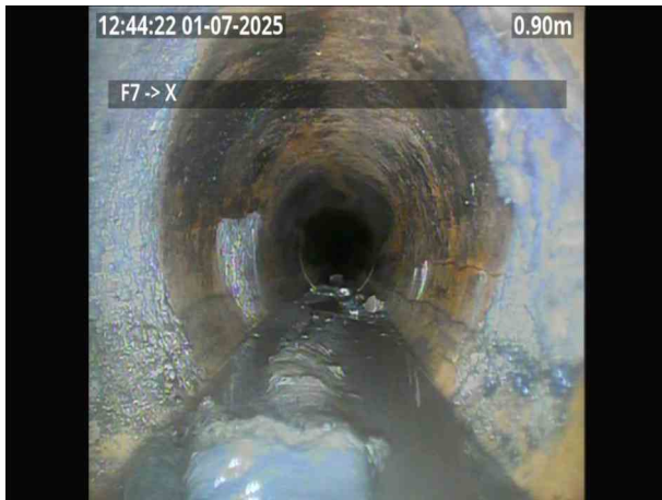
F7X_2cebb3cf-ce4d-48ab-a9af-d0640c6c402a_20250701_125518_818.jpg, 00:00:18, 0.90 m Attached deposits, encrustation at joint from 6 o'clock to 4 o'clock, 10% cross-sectional area loss
