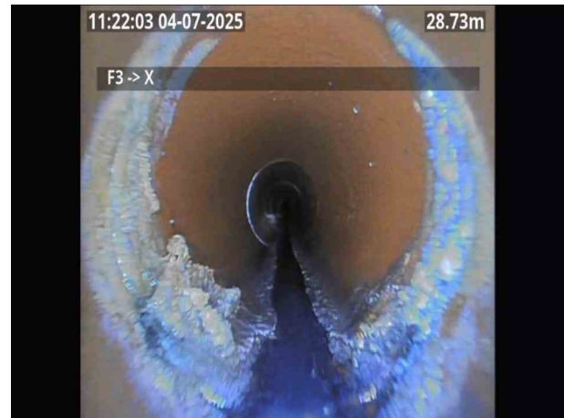
F3X_b7029ac4-ffbb-4223-847e-aea42a170885_20250707_122521_263.jpg, 00:02:54, 28.75 m Attached deposits, encrustation at joint from 2 o'clock to 10 o'clock, 10% cross-sectional area loss
