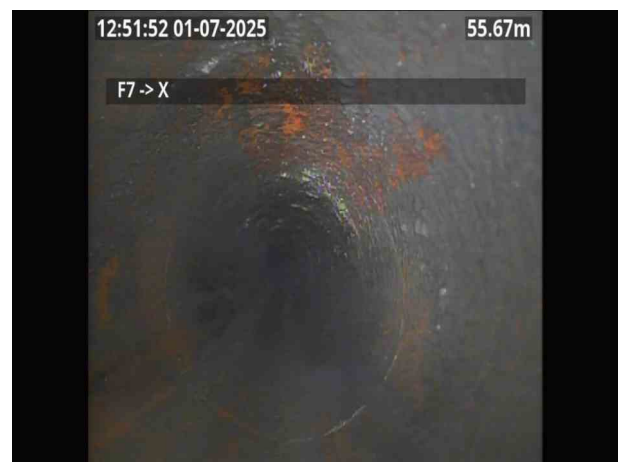
F7X_1ef5af32-a849-4c28-9d9b-125c606dfdfa_20250707_113330_364.jpg, 00:07:25, 55.70 m Crack, circumferential from 2 o'clock to 10 o'clock
