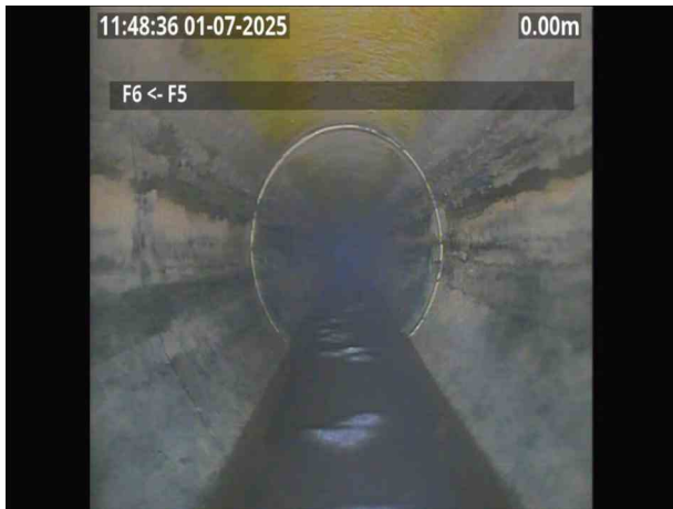
F6X_6f4d11eb-525f-4dc1-817c-110dd92e14c7_20250701_115932_570.jpg, 00:00:09, 0.10 m Fracture, circumferential from 7 o'clock to 11 o'clock
