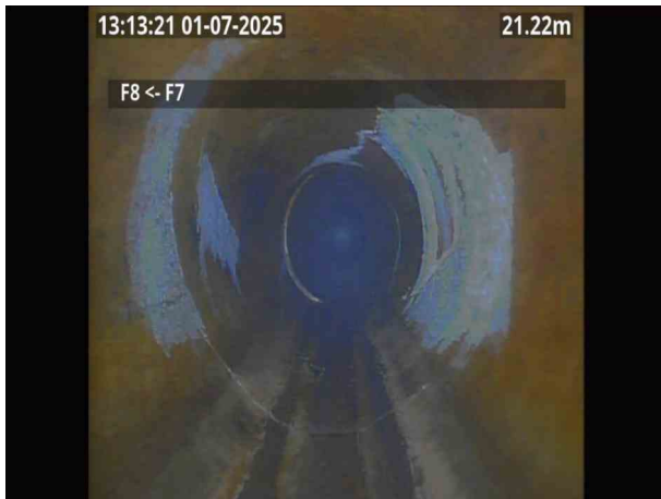
F8X_60b6ea5c-6835-4b66-8df7-946466924d2d_20250707_1 15901_741.jpg, 00:03:07, 21.31 m Fracture, circumferential from 4 o'clock to 11 o'clock
