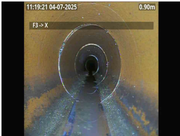
F3X_961426f9-a001-4769-bea9-90aeee7a0536_20250704_13021_277.jpg, 00:00:21, 0.90 m Crack, circumferential from 9 o'clock to 3 o'clock
