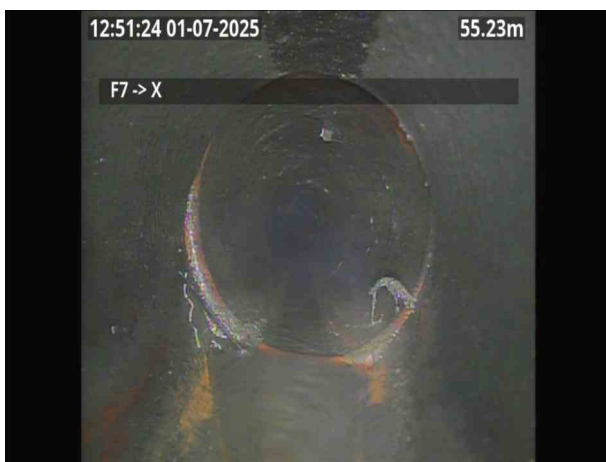
F7X_2b78a31f-4bd2-423a-b797-2f050bc601a7_20250701_130220_558.jpg, 00:06:56, 55.20 m Broken pipe at joint from 5 o'clock to 7 o'clock
