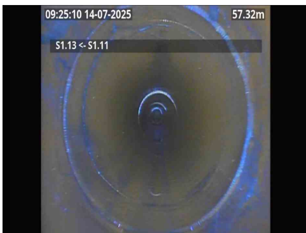
S1.13X_3d42556b-dd6c-4ab5-b3a2-4e8464f05179_20250715_132704_236.jpg, 00:04:13, 57.33 m Fracture, circumferential at joint from 5 o'clock to 2 o'clock
