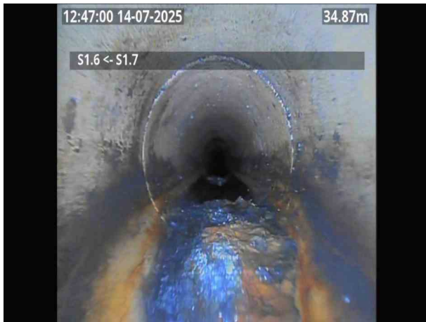
S1.6X_66bce885-8676-48f8-a509-218a3099b25c_20250715_134325_332.jpg, 00:02:42, 34.93 m Settled deposits, hard or compacted, 20% cross-sectional area loss
