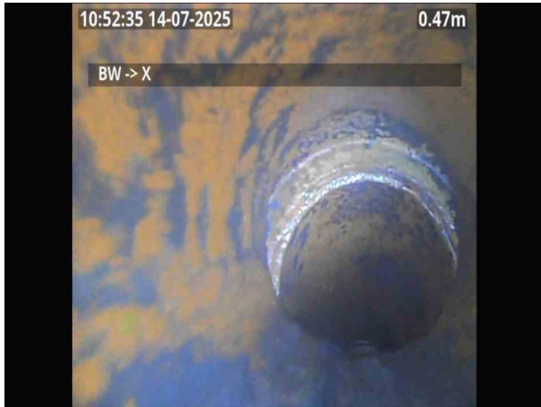
BWX_10a2d309-bf9d-4a8d-950a-84363a479038_20250715_133735_235.jpg, 00:00:21, 0.66 m Joint displaced, large
