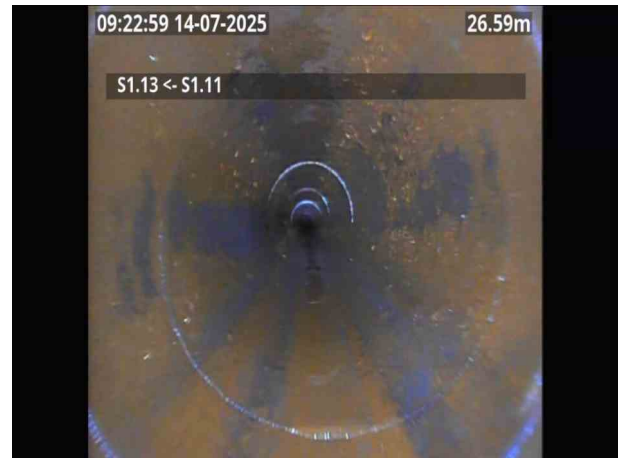
S1.13X_e204bb02-9875-4ed0-a359-01c3a86236f2_20250715_132329_615.jpg, 00:02:03, 26.61 m Fracture, circumferential at joint from 2 o'clock to 9 o'clock
