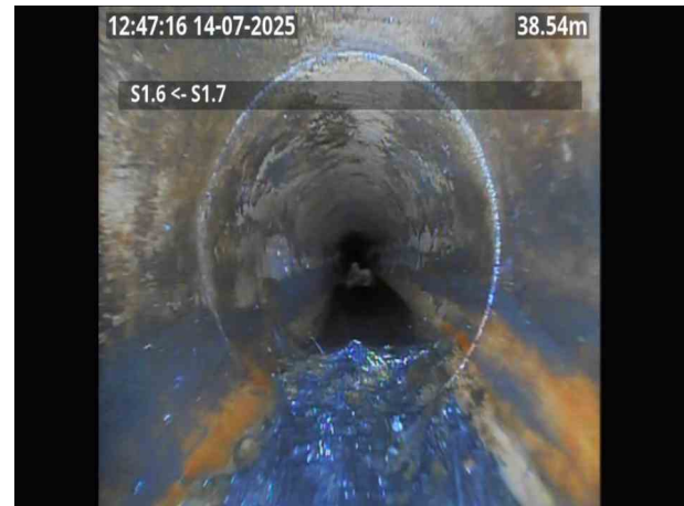
S1.6X_77c98f29-0388-4d0c-83f4-03005816b0a3_20250715_134346_511.jpg, 00:02:58, 38.55 m Settled deposits, hard or compacted, 15% cross-sectional area loss
