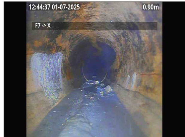
F7X_e866e143-6df4-4900-a2e6-2bbadc6be201_20250701_125533_625.jpg, 00:00:26, 0.90 m Fracture, longitudinal at 3 o'clock
